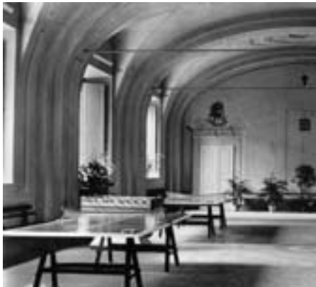
The Scuola: Aula Magna and after restoration
