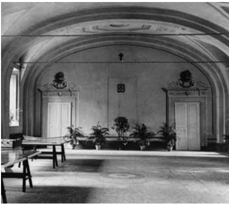
The Scuola: Aula Magna before and after restoration
